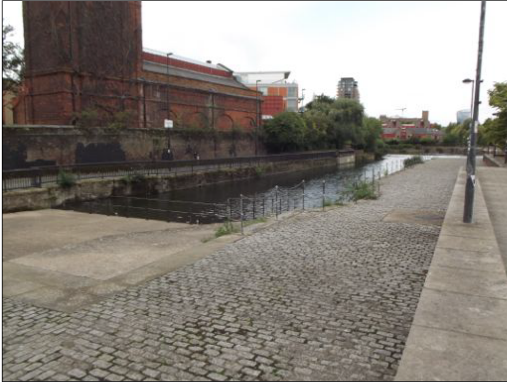
Figure 1: Photo of the existing site looking west
